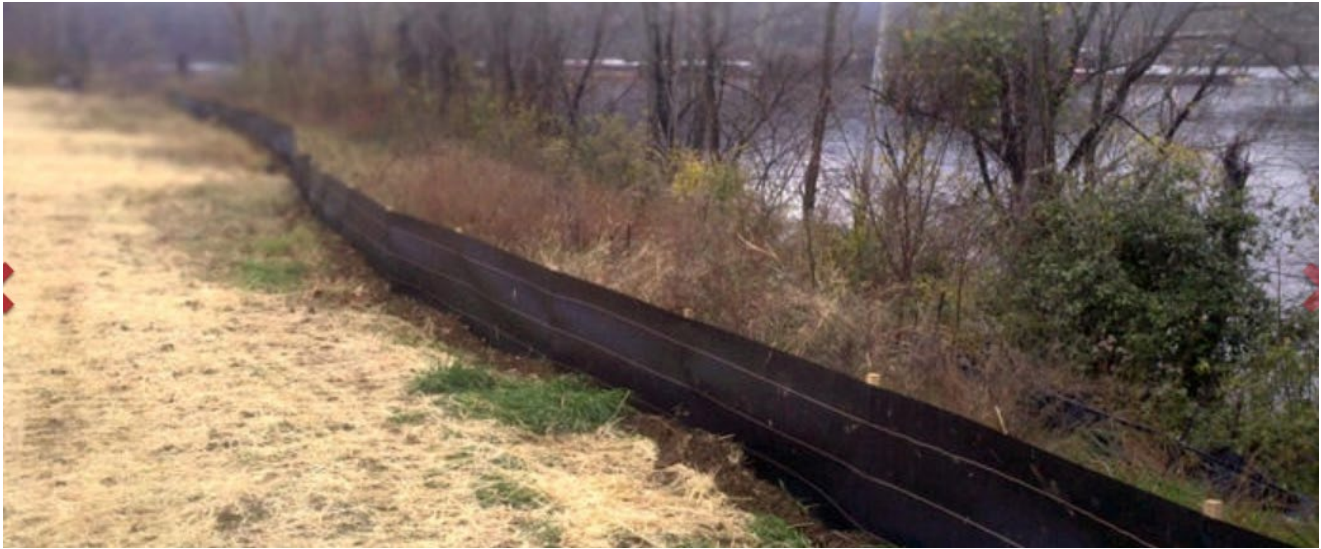
Figure 4.4: Typical Silt Fence 2
